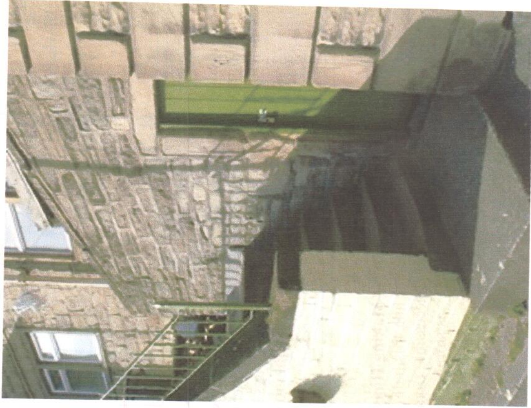
Figure 9. LEFT - Stone doorway with recessed frame, part of the original construction of Litt House. RIGHT - This doorway is inside the access underneath the old stone steps.
