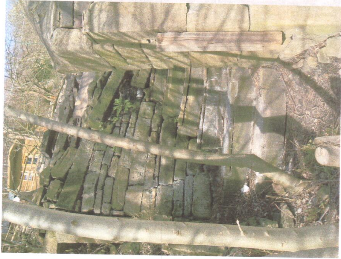
Figure 15. LEFT- The rear wall of the old road level beer garden, stonework dating probably from the 1500s and being the back wall of the narrower building. RIGHT - these stone steps lead up to the left of the wall, and were part of the access from the road to the cottages of Solomons Backside.
